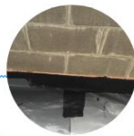
7 Sealing "Film-11" Membrane at Foundation Perimeter
