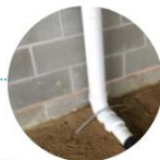
2 Installing Vent Risers
