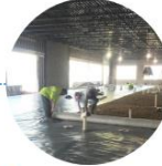
4 Rolling Out "Film 11" Membrane
