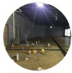
1 Installing Sub-membrane Vent Runs
