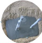
3 Installing "Grout Blocks" at Nested Utility Penetrations
