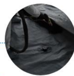
8 Sealing "Film-11" Membrane Overlap Boundaries
