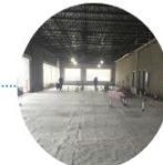
14 Geo-Seal Bond Protection Layer Installed
